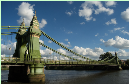
Hammersmith Bridge (Londres)
